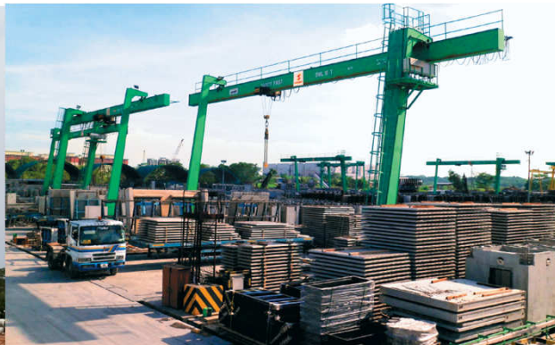
Precast Yard in Singapore
